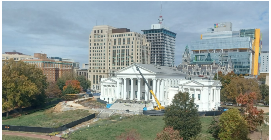
Virginia's State Capitol Undergoing renovations.
